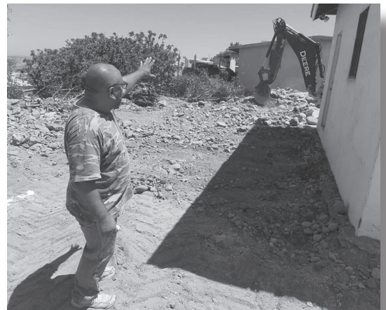
Leveling the ground for the new addition
