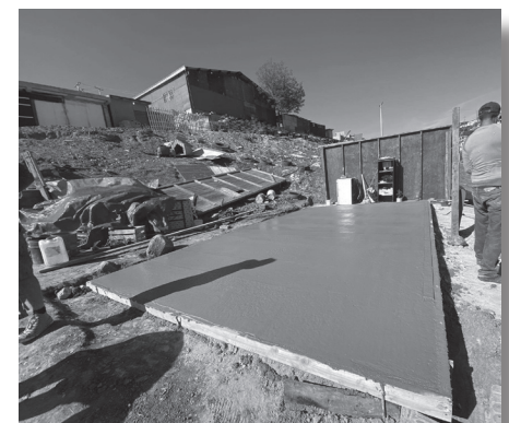
Having a firm foundation is always important.
